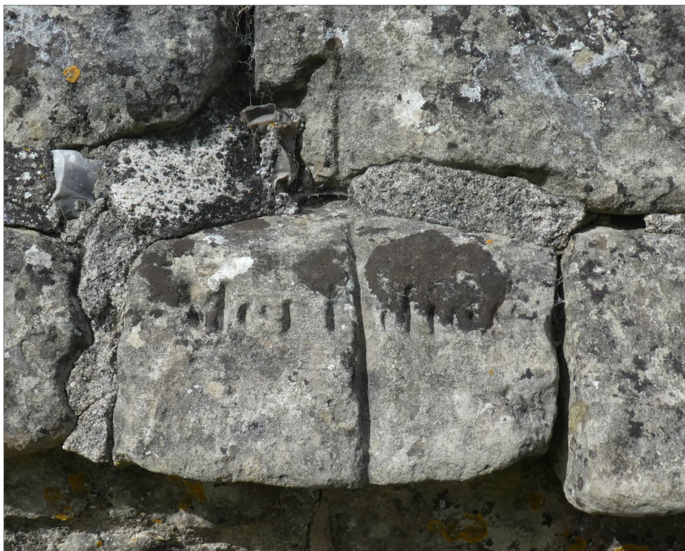
The meridian mark, on the wall near No. 28 The Close
