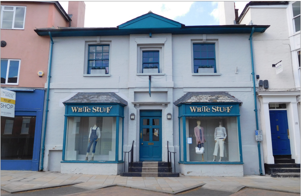
Former Police Station in New Canal
