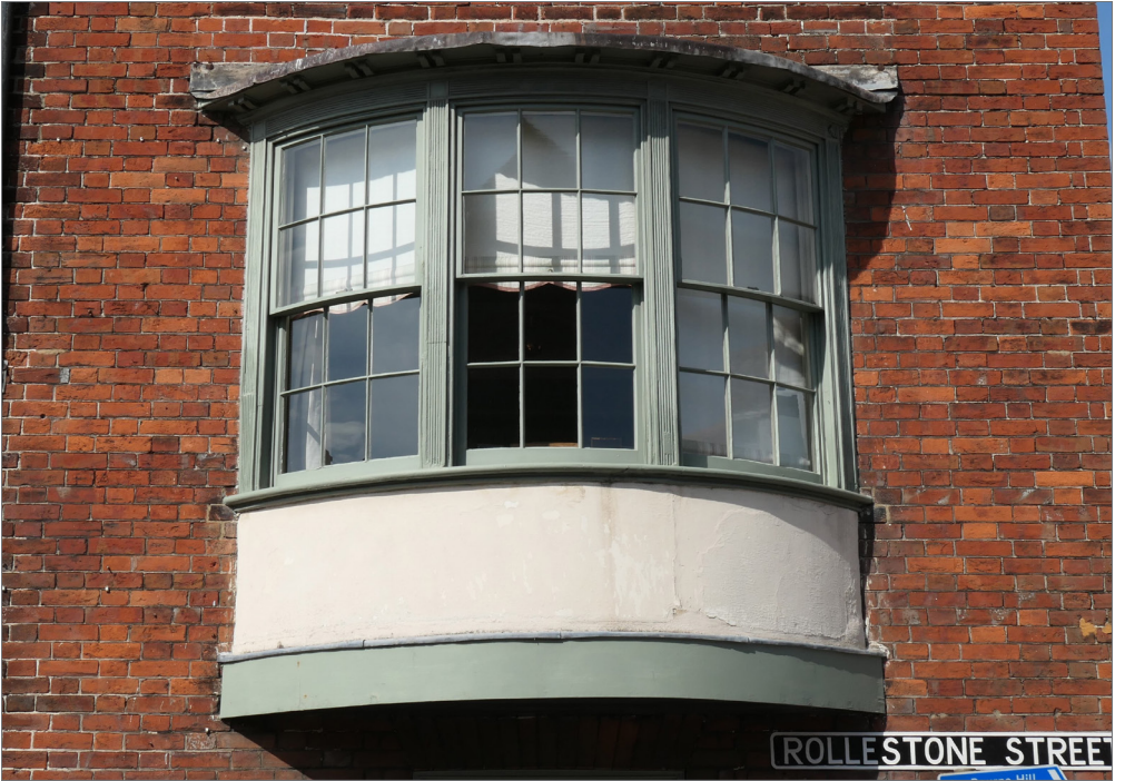
Oriel window in Rollestone Street
