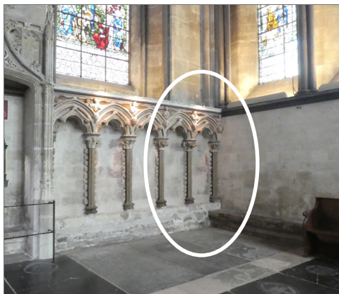
Base of tower staircase viewed from inside at corner of the Morning Chapel
