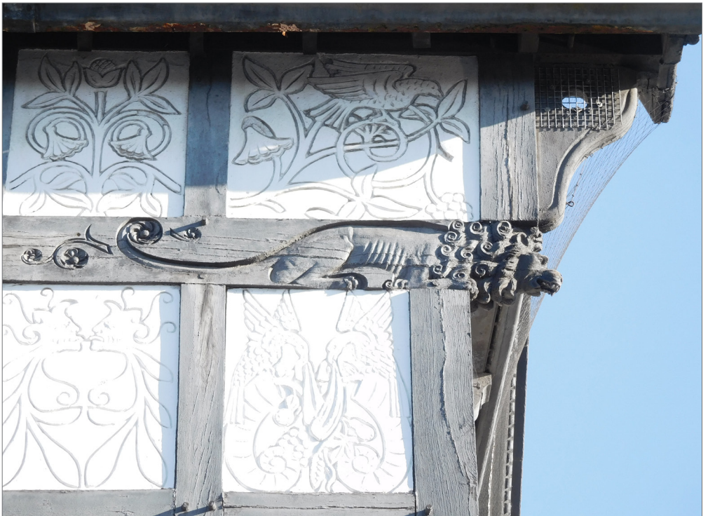
Plaster panels at Cross Keys House, Queen Street (see p.21)
